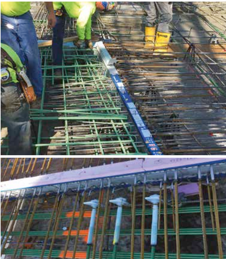
Underside of slabs reveal The Spark's post-tension concrete construction supporting 10 ft (3 m) cantilevered balconies.
